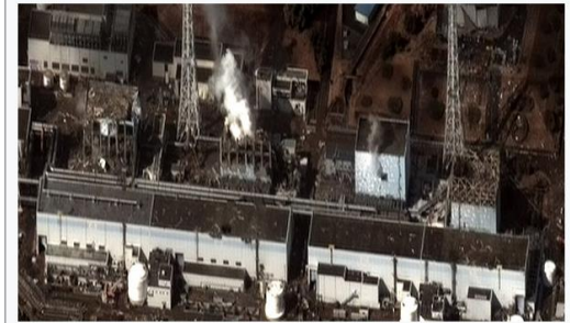
Image on 16 March 2011 of the four damaged reactor buildings. From left to right: Unit 4, 3, 2, and 1.
